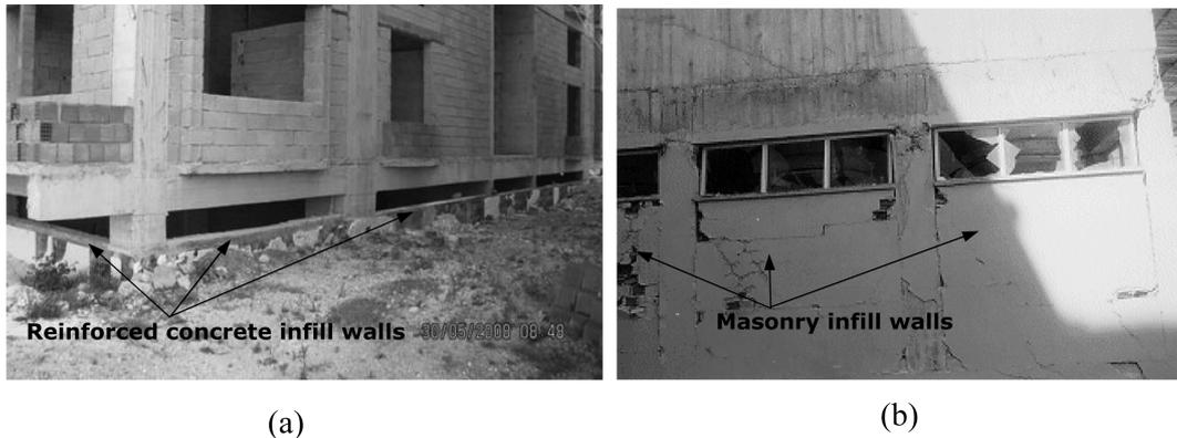
Fig. 1 Infill wall under the band window (a) reinforced concrete, (b) masonry
