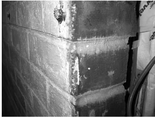
Fig. 20 Cracking of the conventional BV at the bed joint
