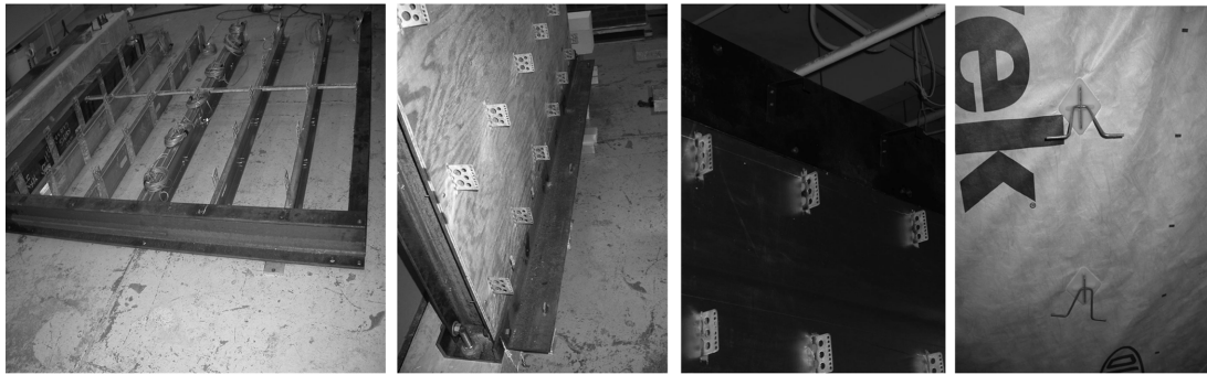
Fig. 4 Attachment of shear connectors to the studs and wall assembly
