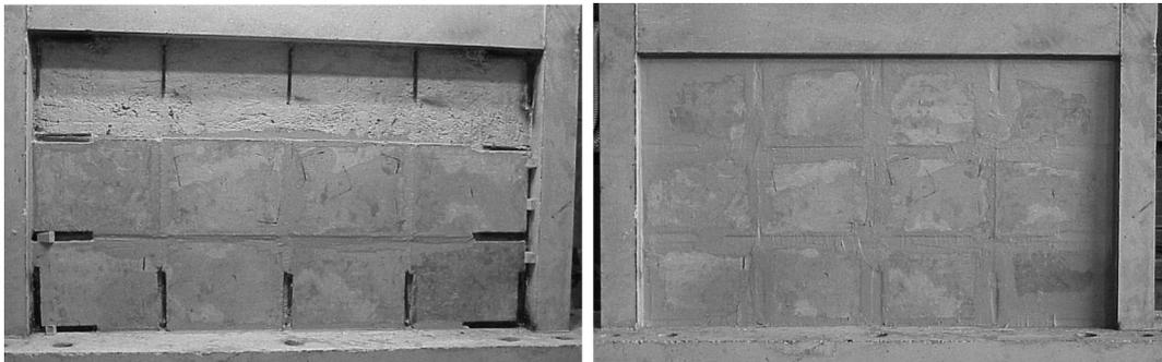
Bonding panels on to the hollow brick infill – filling the gaps with epoxy
