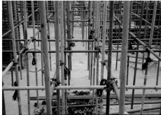
Fig. 7 Shore load measurement
