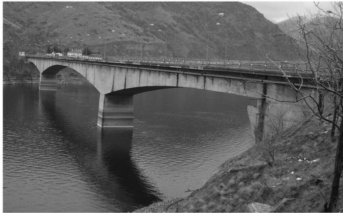
Fig. 1 Kömürhan Highway Bridge constructed with balanced cantilever method
