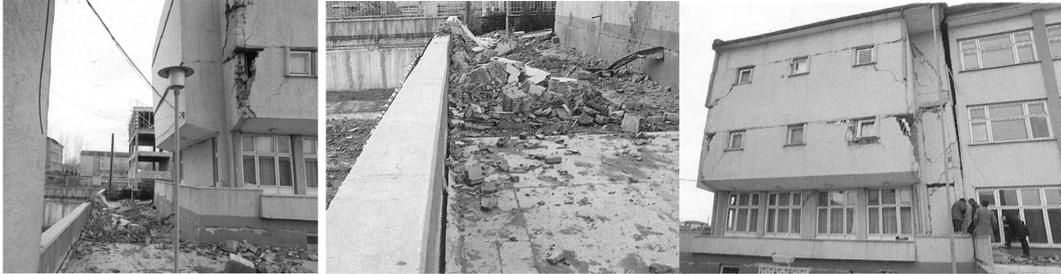
Fig. 1 A real example of retaining wall damaged in Erzincan Earthquake
