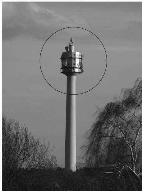
Fig. 1 Possible tuned mass dampers location in a tall tower
