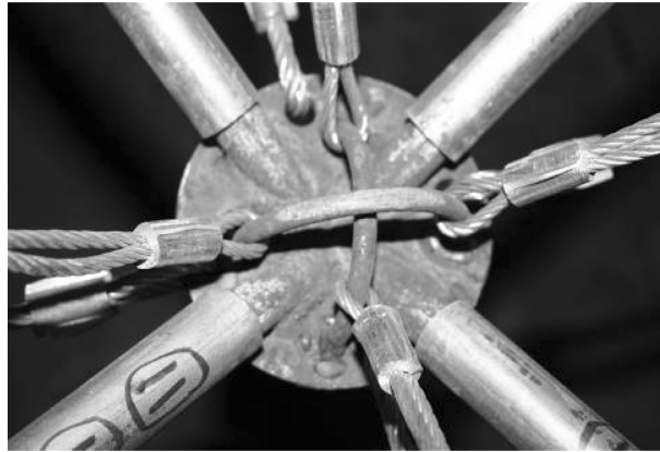
Fig. 3 Detail of central bottom joint
