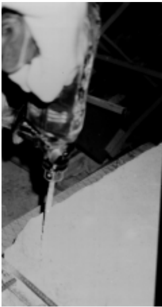
Fig. 7 Drilling of holes in the beam
