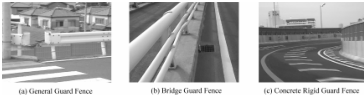
Fig. 3 Existing guard fences
