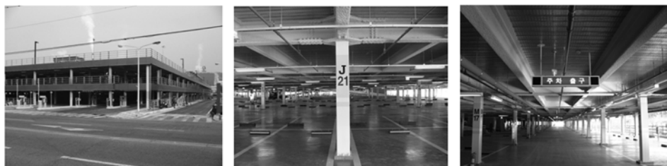
Fig. 4 Square CFT columns without fire protection applied to the parking garage of Samsung Electronics
