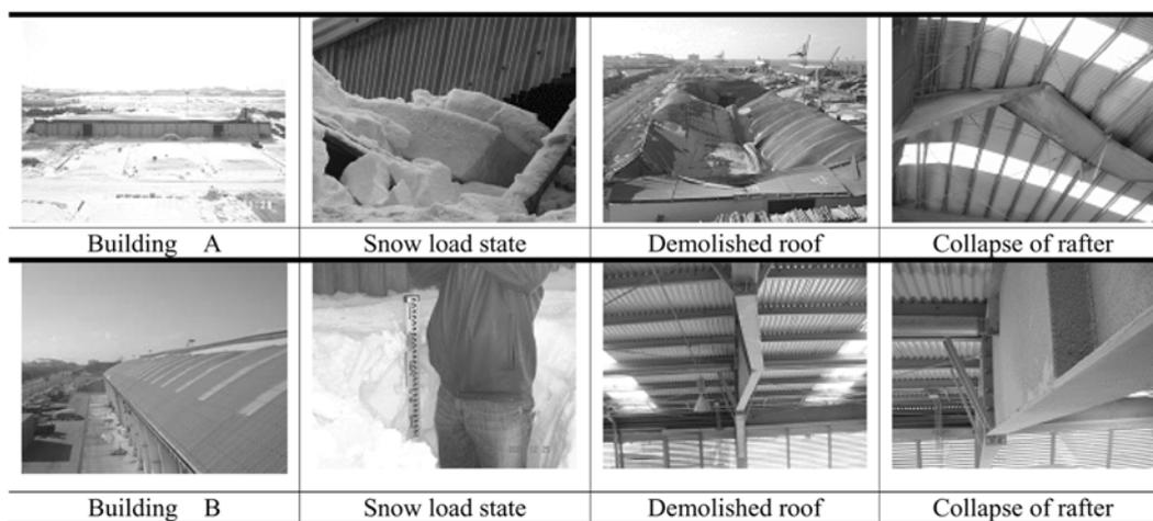
Fig. 1. Warehouse building collapse
