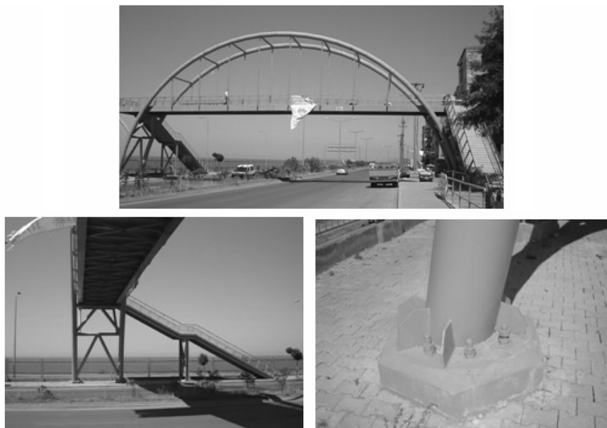
Fig. 1 Some views of the arch type footbridge
