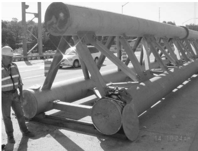
Fig. 1 Tri-chord overhead highway sign structure
