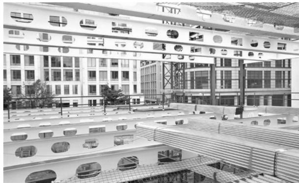
Fig. 2 Fabricated beam with elongated and rectangular openings
