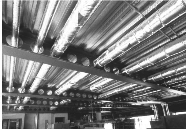
Fig. 1 Cellular beam with regular openings for services
