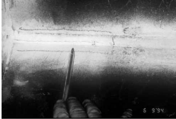
Fig. 7 Hydrogen cracking of ultra high strength steel
