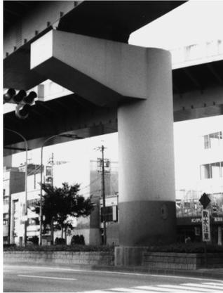
Fig. 1 An eccentrically loaded steel tubular bridge pier
