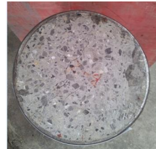
Fig. 7 Crack of the concrete
