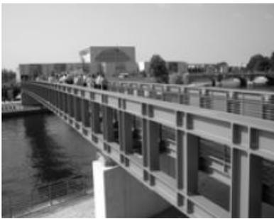
Fig. 4 Vierendeel frame used in the construction of a bridge
