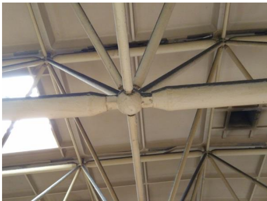
Fig. 2 Bolt-sphere joint entities
