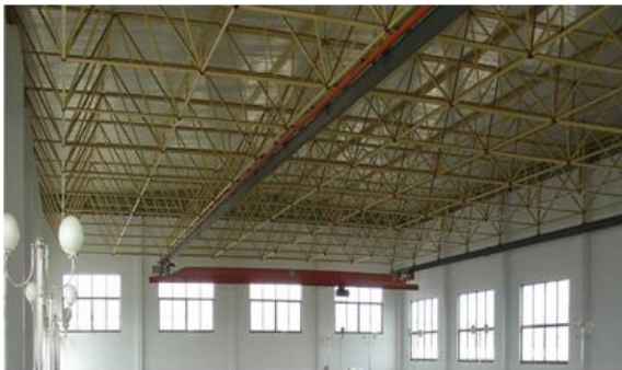
Fig. 1 Grid-structure industry workshop with hanging crane
