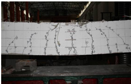
(c) Crack distribution
