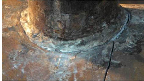
Fig. 7 Failure mode of un-stiffened specimen
