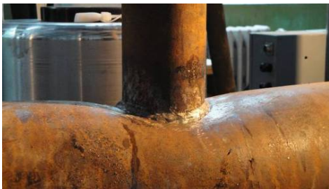
Fig. 5 Local buckling of un-stiffened specimen
