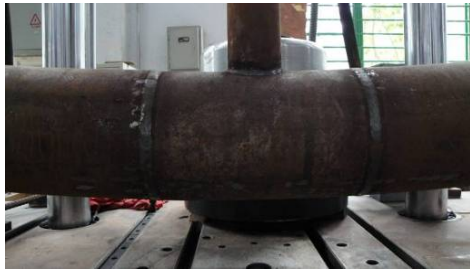
Fig. 8 Yielding of the stiffened specimen
