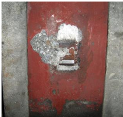
(a) Fractured channel in slab
