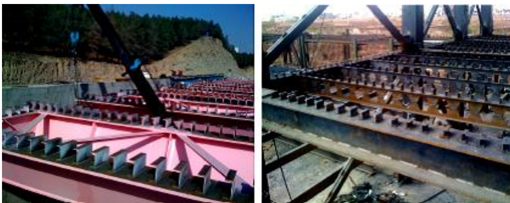
Fig. 2 Application of channel shear connectors in bridge and building
