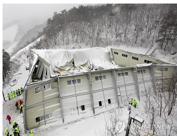
(a) Collapse of roof
