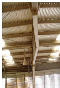
(b) Lateral torsional buckling
