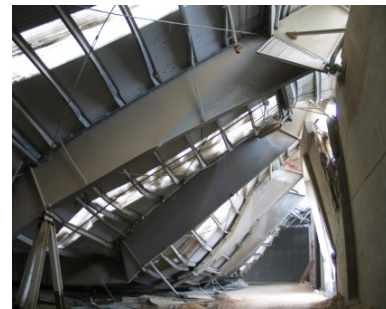
(c) Deformation of rafter
