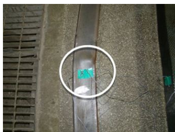
(h) Local buckling at mid-part (LN-20-0L)
