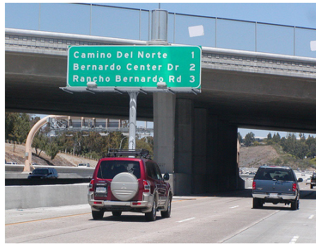
Fig. 2 Tubular members in overhead traffic signs
