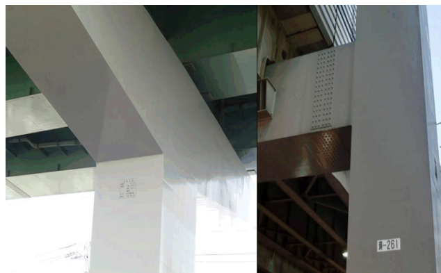
Fig. 1 Beam-column connections in steel piers with very small fillet radius
