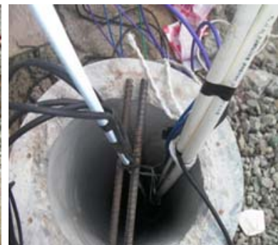
(c) Attachment of sensors
