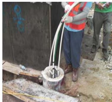
(b) Installation of GHE into piles
