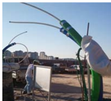
(e) Heat conservation of pipes
