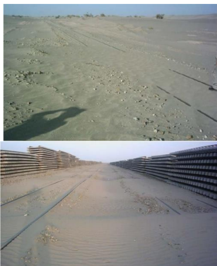
Fig. 1 The tracks contaminated significantly with sand (Iranian eastern railway network)
