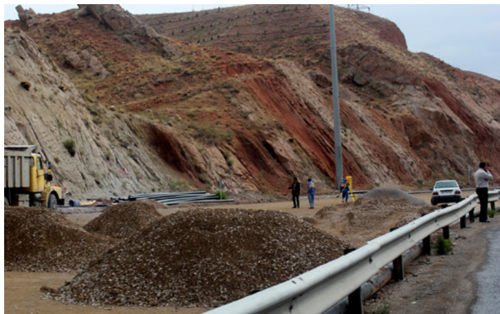
Fig. 3 Treatment of marls in the “Pasdaran highway” of Tabriz
