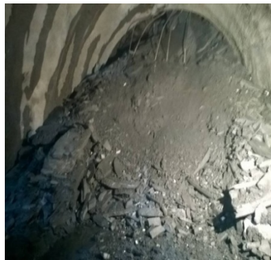
Fig. 6 Collapsing of tunnel
