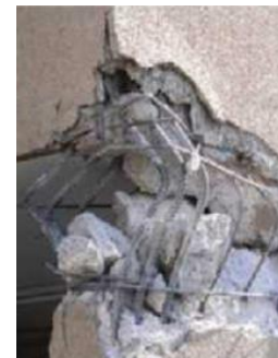
(b) Fracture and buckling of reinforcement in the wall
