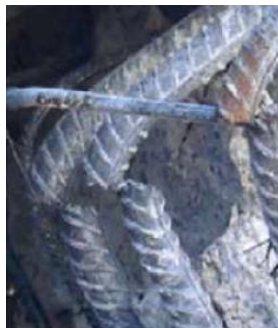
(b) Fracture and buckling of reinforcement in the wall
