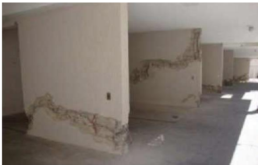
(a) Overall damage in the first-story shear walls
