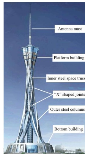
Fig. 1 Structural configuration of Henan tower
