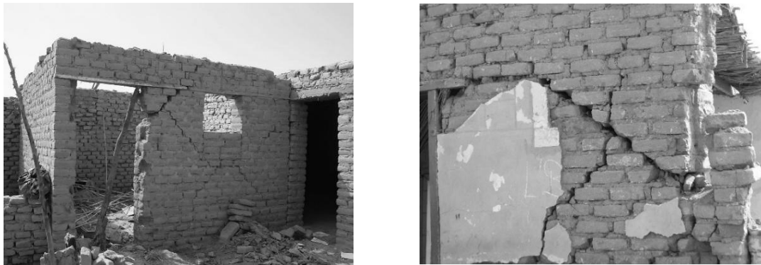
Fig. 2 Typical in-plane damage in adobe walls.
