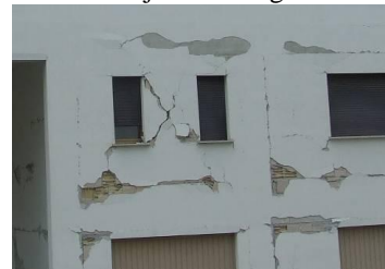
Fig. 1(b) Damage mechanism due to diagonal (stairstep) cracking along with horizontal bed joint sliding
