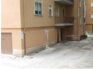
Fig. 2(a) Incipient out-of-plane collapse of the external panel of a masonry infill
