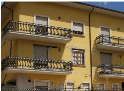
Fig. 1(a) Damage mechanism due to separation of the infill panel from the structural frame
