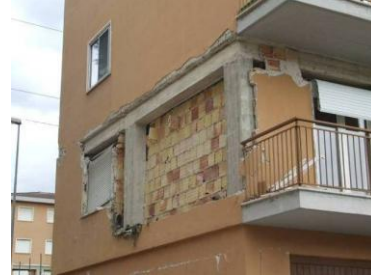
Fig. 2(b) Ejection of the external panel and incipient out-of-plane collapse of the internal panel of a masonry infill
