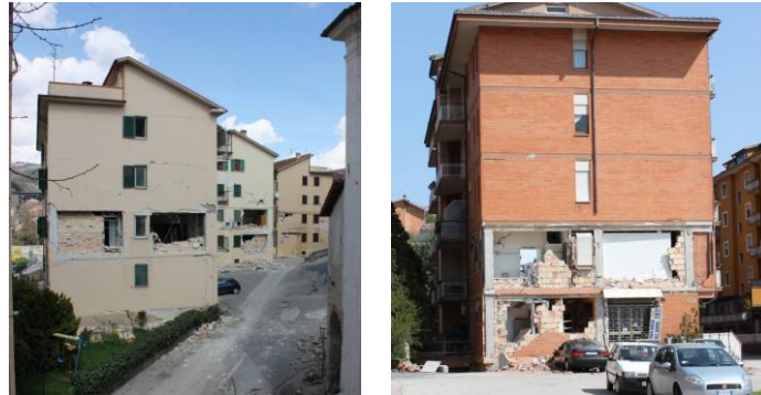
Fig. 11 Examples of damage/collapse of masonry infills typically placed at the lower storeys
