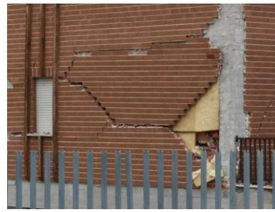
Fig. 1(b) Damage mechanism due to diagonal (stairstep) cracking along with horizontal bed joint sliding
