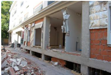
Fig. 3(a) External collapse of infill panels in RC building
