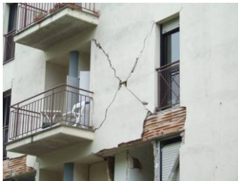
Fig. 1(c) Damage mechanism due to tension stress across the panel diagonals
