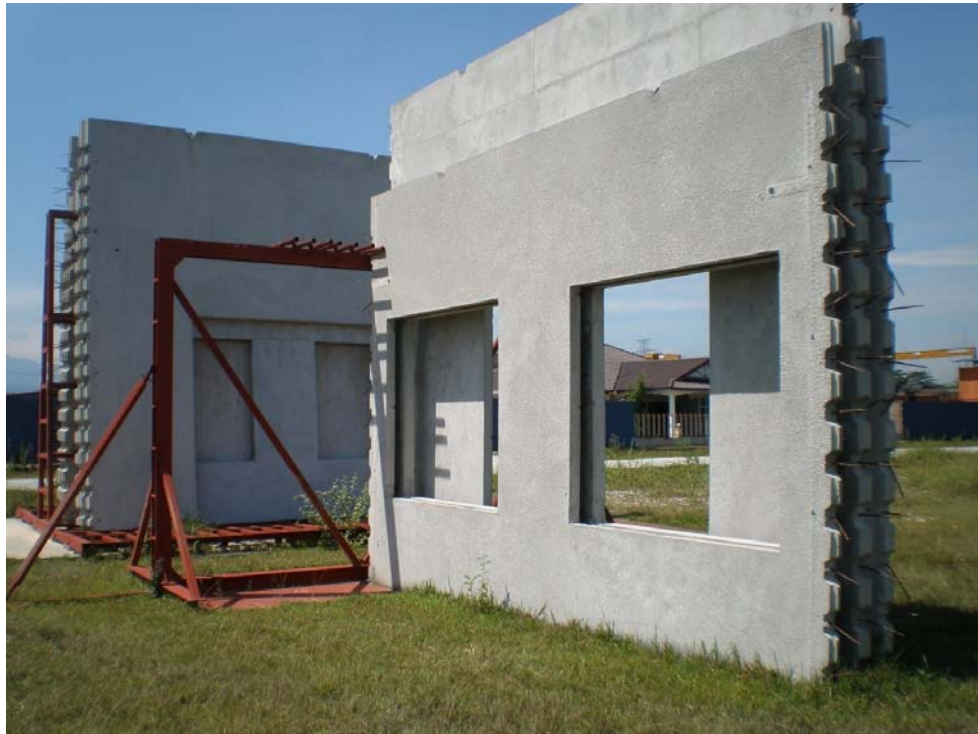
Fig. 2 Panels of HC precast wall system
