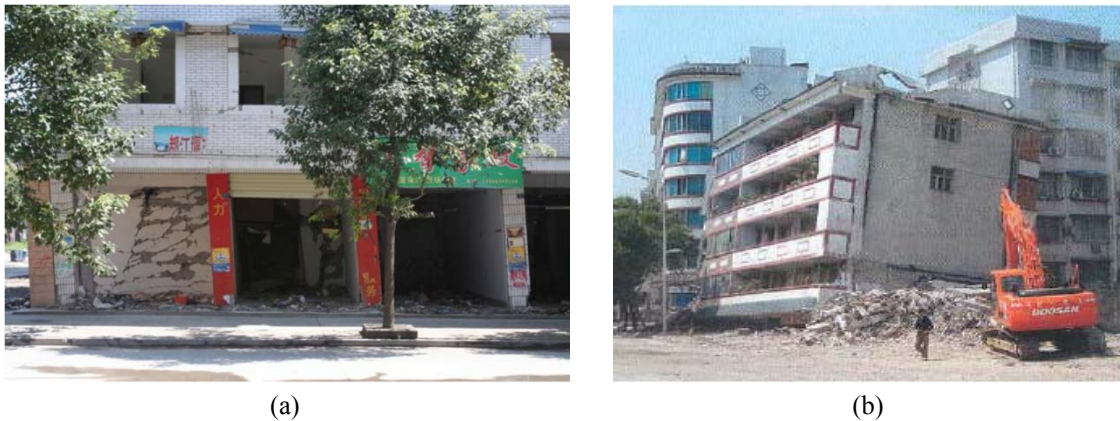
Fig. 1 Damages to masonry buildings in 2008 Sichuan Earthquake: (a) significant drift concentration at the first storey and (b) soft-storey failure at the first storey (China Academy of Building Research 2008)
