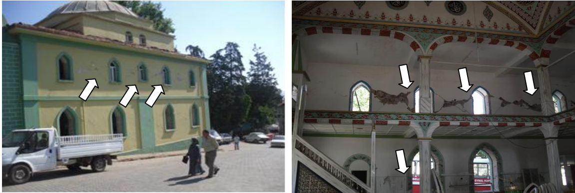
Fig. 7 Shear cracks on the load carrying walls of Halil Aga Mosque
