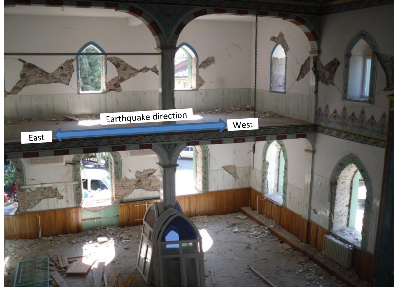
Fig. 11 Shear cracks on the façade of the masonry mosque
