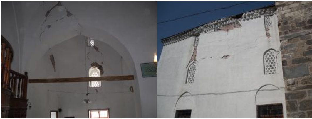
Fig. 6 Severely damage to unreinforced masonry mosque (Ulu Mosque) and example of out-of-plane damage
