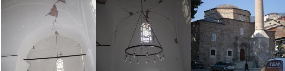
Fig. 5 Shear cracks on the load carrying walls of Halil Aga Mosque
