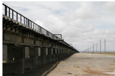
Fig. 1 Photo of a dry bridge along the Qinghai-Tibet Railway
