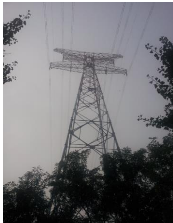
Fig. 4 Practical graph of suspension-type tower
