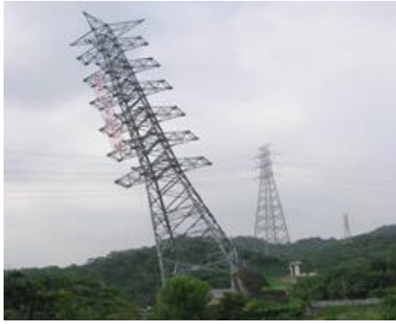
Fig. 2 The collapse of transmission tower in the Chi-Chi earthquake
