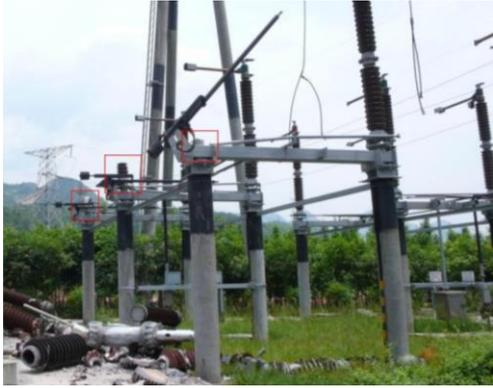
Fig. 1 Failure of cylindrical porcelain equipment in a 220kV substation after 2008 Wenchuan Earthquake (Xie 2013)
