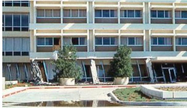
Fig. 1 Soft storey due to elimination of shear walls in ground floor of the Olive View medical center in the 1971 San Fernando earthquake (Arnold 2006)
