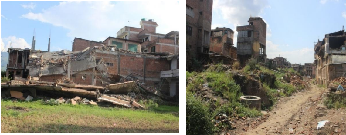
Fig. 10 Damage in RC structure and a completely collapsed neighborhood in Bhaktapur
