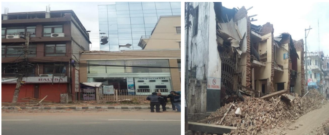
Fig. 14 Toppled parapet wall of RC building and out of plane failure of masonry structure in Jawlakhel
