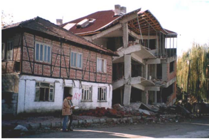
Fig. 3 View of traditional himis and reinforced concrete building after the 1999 Izmit earthquake in Turkey
