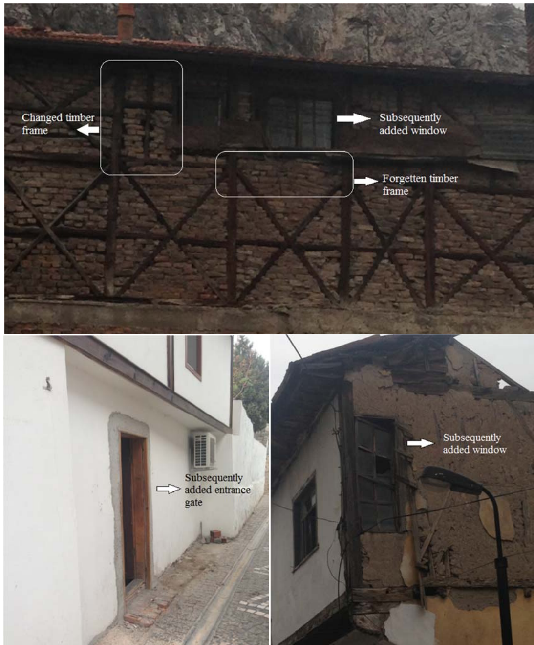
Fig. 4 Non-engineering additions and changes (Photographs by the authors)
