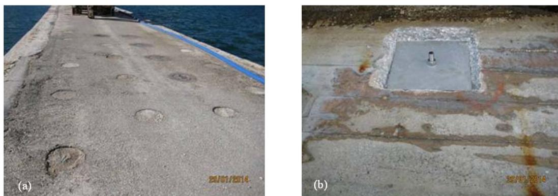
Fig. 14 (a) Group of micropiles drilled from the bridge deck (b) Steel plate embedded in the lateral façades of the bridge for anchoring the stainless steel tendons
