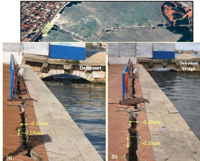
Fig. 17 Recorded failures adjacent to the “De Bosset” bridge; permanent lateral displacement of the quay wall and settlement of the backfill induced by (a) the first M6.1 earthquake event of 26/01/2014 (13:55GMT) and (b) the second M6.0 earthquake event of 03/02/2014(03:08GMT)
