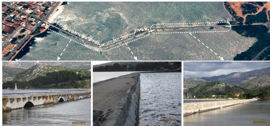
Fig. 16 In-situ inspection of the rehabilitated “De Bosset” bridge after the two major Cephalonia earthquakes of 01/26/2014 and 02/03/2014, revealing no damage or visible defects at the bridge structure
