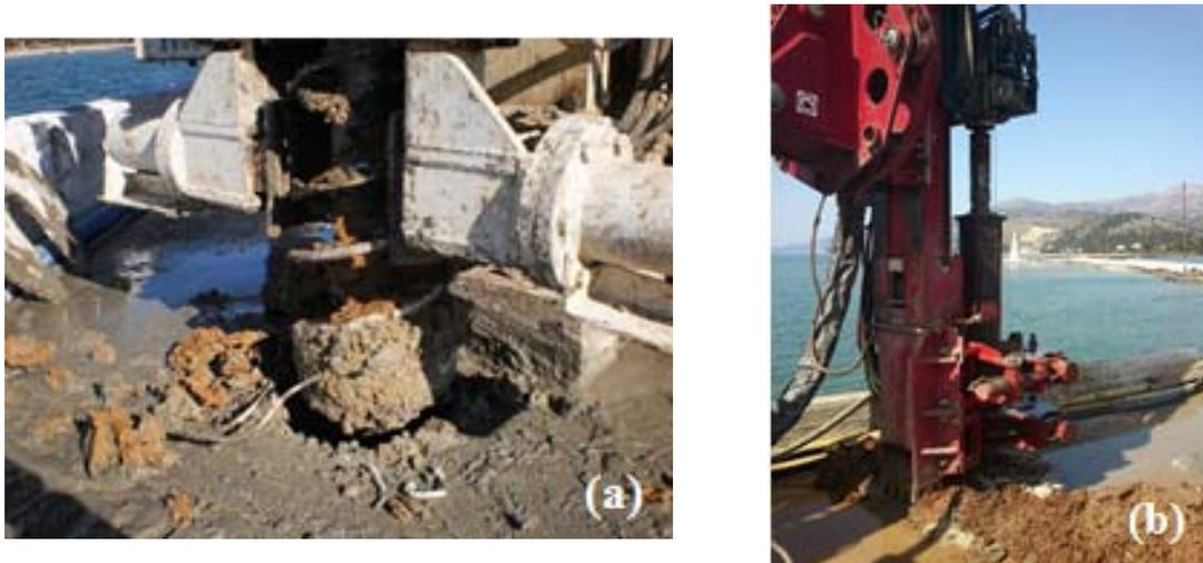
Fig. 13 (a) Filling material of the bridge composed of soil, sparse steel bars and debris that was revealed during restoration works (b) Steel tubes embedded consecutively to prevent debris fall inside the borehole during the drilling of the micropiles
