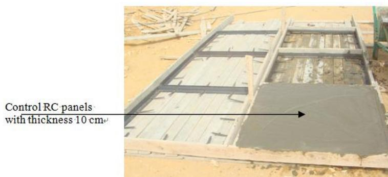
Fig. 1 Assembled reinforced concrete (RC) panels (Control RC panel)
