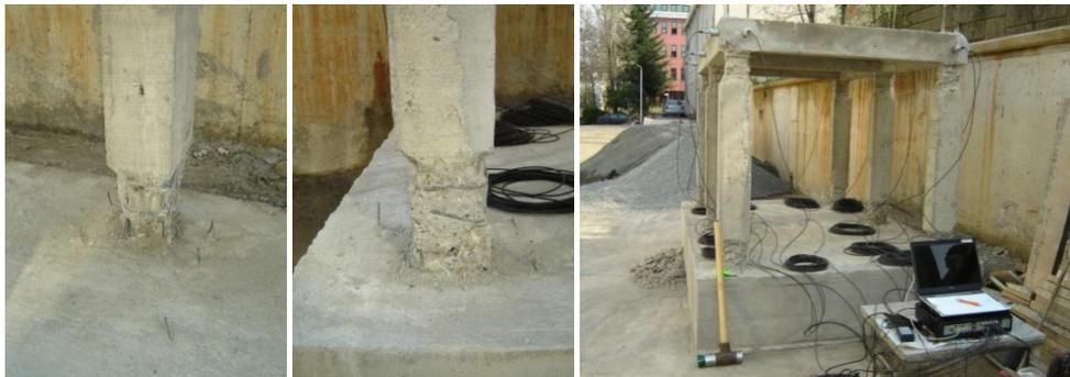
Fig. 13 The damages on the lower parts of the column and measurement system
