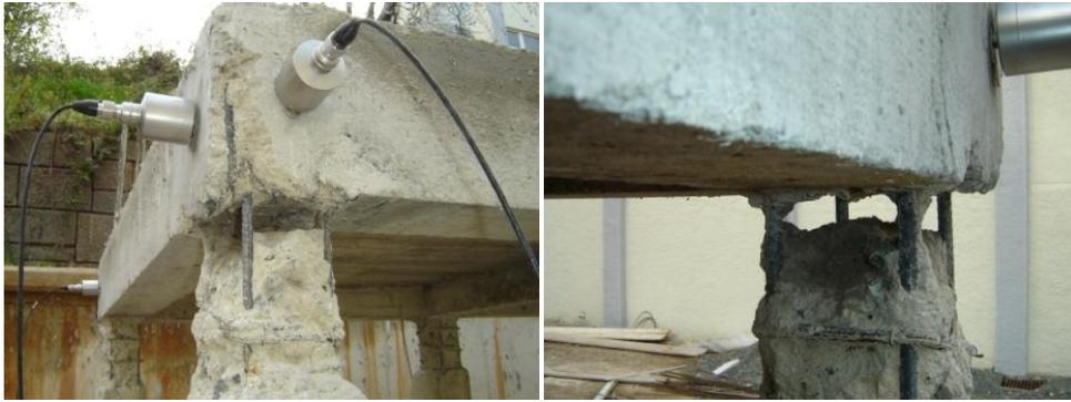
Fig. 15 The damage case for the core-concrete on the upper part of a corner column
