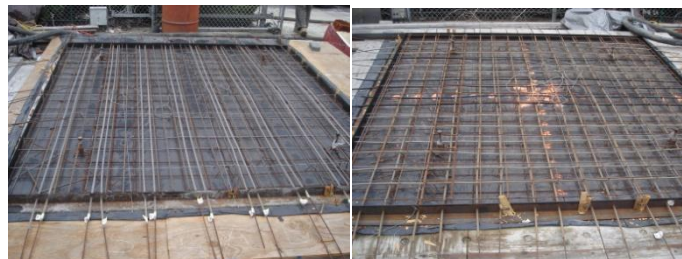
Fig. 2 Tendon layout for one-way and two-way slabs
