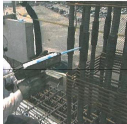
(c) Grout work
