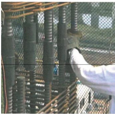
(b) Tightening the mechanical sleeve
