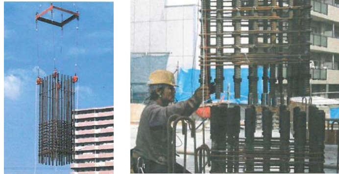
(a) Erection of pre-fabricated reinforcement cage
