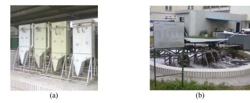
Fig. 3 Pictures of (a) single rotating wheel lifting bioreactor; and (b) rotating wheel bioreactor combined with hollow fiber filtration system
